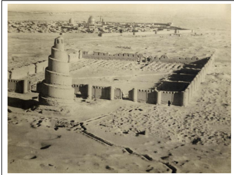
Aerial View of the Milwaya and the City Of Samarra 1920
