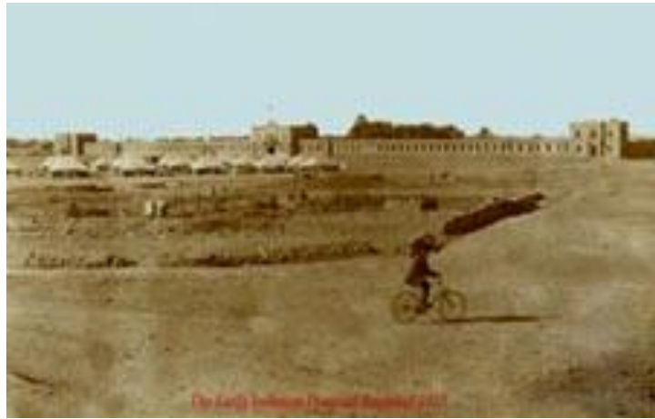
Tents Isolation hospital Infront of Quarantine Building. North of Bab Mudhum
